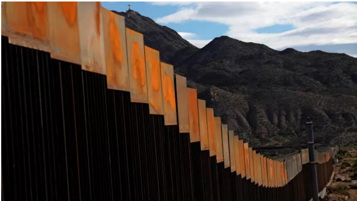
Source – Reuters, a newly-built section of the US – Mexico border wall at Sunland Park, opposite the Mexican border city of Ciudad Juarez
